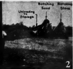
2.—Barber-Greenes with strike-off hoppers ran 824 feet of 16-foot road in one day on this job. Shown on page 7 of "Contracting with Barber-Greenes."
